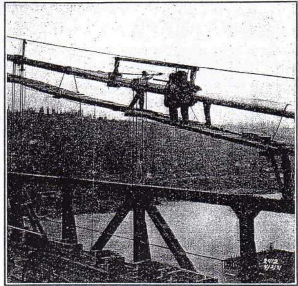
WRAPPING OF THE MAIN CABLE.
