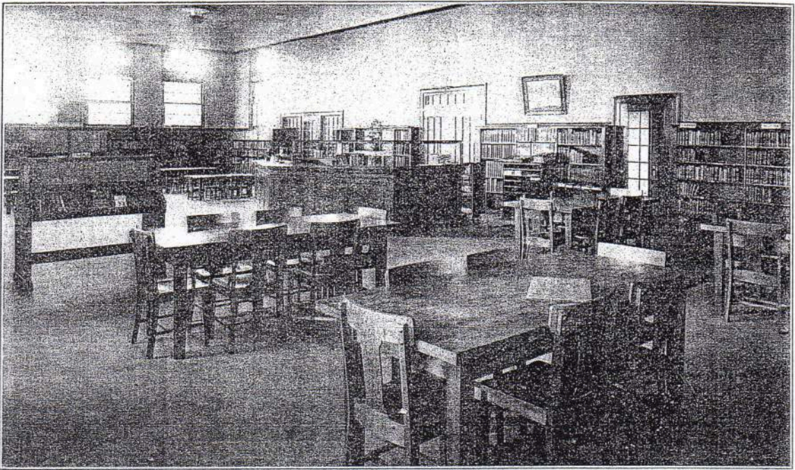
INTERIOR VIEW OF BEAUTIFUL ST. JOHNS LIBRARY
